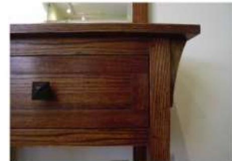
All the hardware use is hand cast and the frame is built with traditional mortise and tenon joinery.
