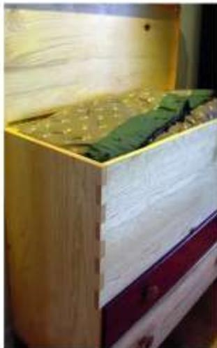
The chest's sides and front are joined with a typical box joint. The chest is lined with cedar.
